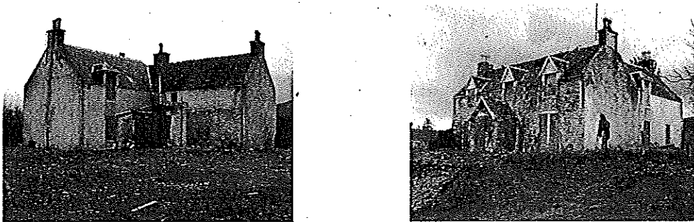
Figs 8 & 9 : existing derelict dwelling on eastern boundary
